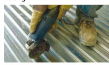
To cut LEWIS<sup>®</sup> sheets to size a carborundum disc cutter can be used. Cut outs can also be made this way or with the use of a suitable jig saw. Holes through a completed LEWIS<sup>®</sup> floor can be made with a core drill.
