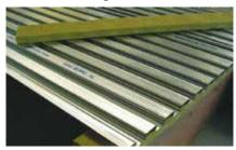
Timber or steel construction - place LEWIS® 25/20 Resilient strips directly on top of new or existing beams or directly onto an existing or new timber floor deck. When laying acoustic strips on a timber deck: place the LEWIS® Resilient strips at between 500 - 600 mm centres.
