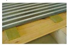
Please note: A resilient strip must always be placed directly under any lengthwise overlaps of the LEWIS® deck, overlaps should be a minimum 100 mm. Around the perimeter of each dwelling or room LEWIS® 20/15 Flanking strips must be used to create complete isolation of the floating floor from the supporting structure and party walls. Avoid any potential for "sound bridging" by wrapping all pipes and voids with LEWIS® 20/15 Flanking strip.
