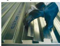
Overlaps should not be limited to the side flanges. In order to make the LEWIS® floor less vulnerable to site foot traffic (vibration movement), it is necessary to include part of the profile itself in the overlap.
